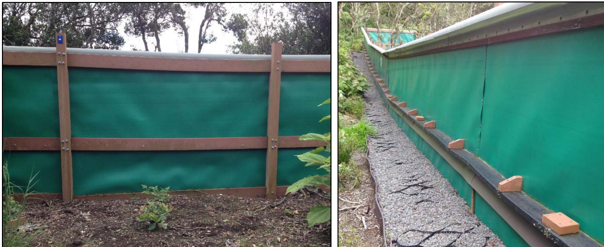
Figure 5. Palikea North enclosure design: wall frame inside of enclosure (left), and outside wall with E. rosea barrier, rat hood, and erosion control (right).
