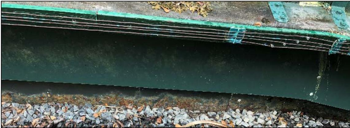
**Figure 28.** Corrosion at base of Palikea South enclosure wall
