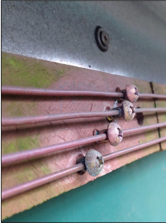
**Figure 25.** Copper wires held in place by stringing through holes drilled in brass screws.
