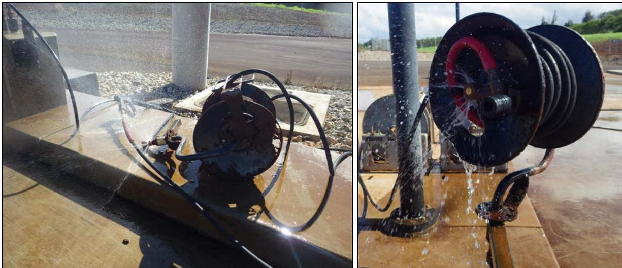
**Figure 9.** Left: this hose reel is detached from its mount and now sits on the ground, the reel is rusted through, and water leaks from all connecting points. Right: while still on its mount, this hose reel leaks prolifically.
