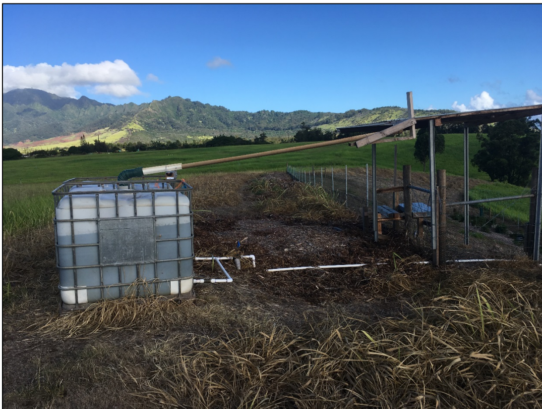
Figure 4. Water catchment system at Kahua site.
