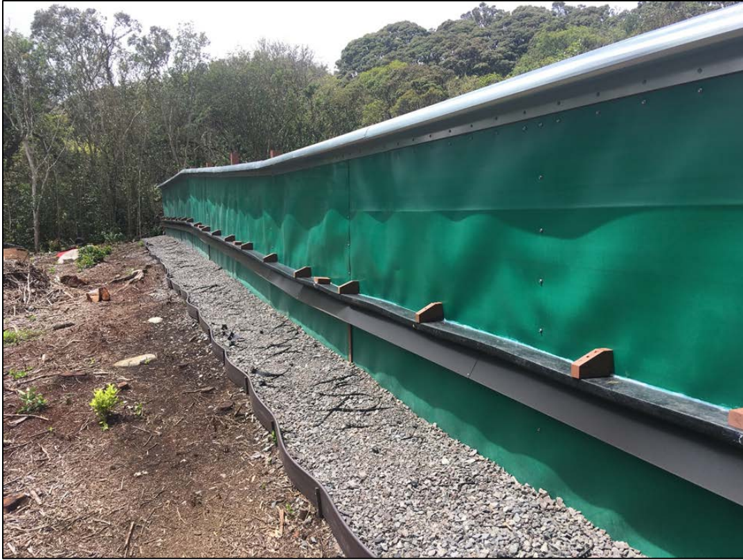
Figure 18. Palikea North snail enclosure wall with E. rosea barriers, rat hood and erosion control
