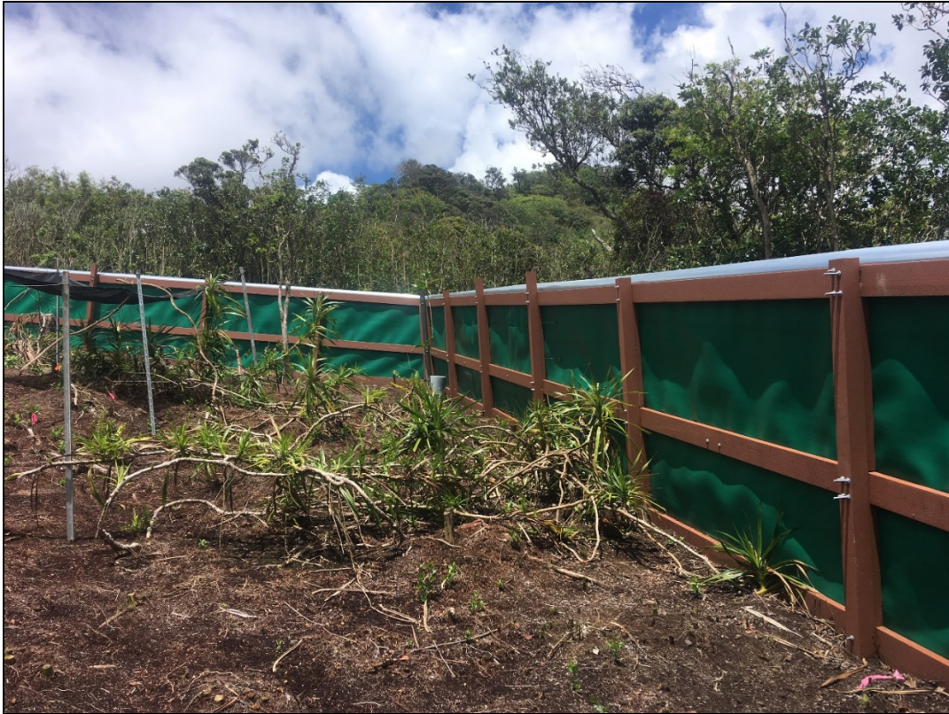
Figure 17. Palikea North snail enclosure wall frame, inside of enclosure
