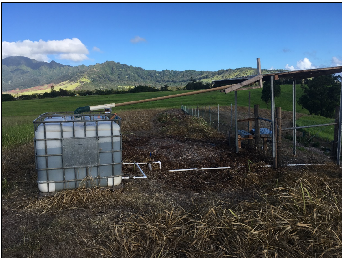
Figure 4. Water catchment system at Kahua site.
