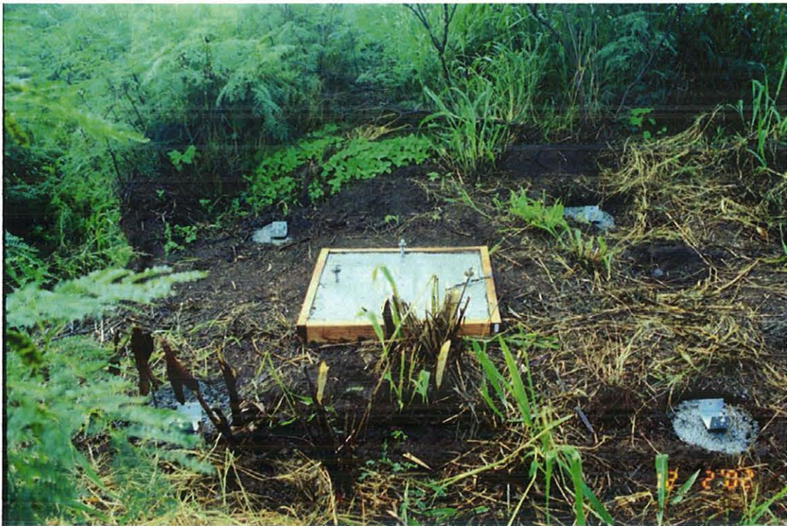
Figure 72. Large Equipment Pad and Shelter Footings on Bank, for Flow Meter.
