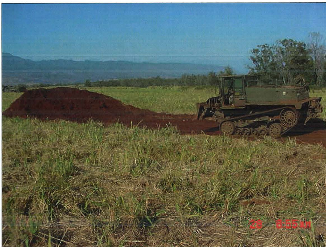
Figure 21. A 'Deuce' Beginning Excavation of TOC Surrounding Berm. Viewed to West.
