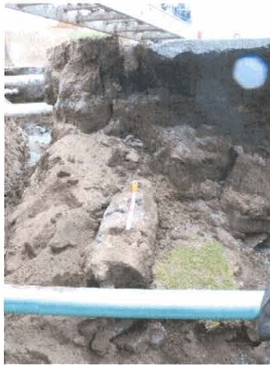
Plate 87. This is a view of the concrete pipe base found during excavation of Septic Tank #14. The scale is 0.50m long. Note the mold of the feature in the wall below the horizontal ladder.
