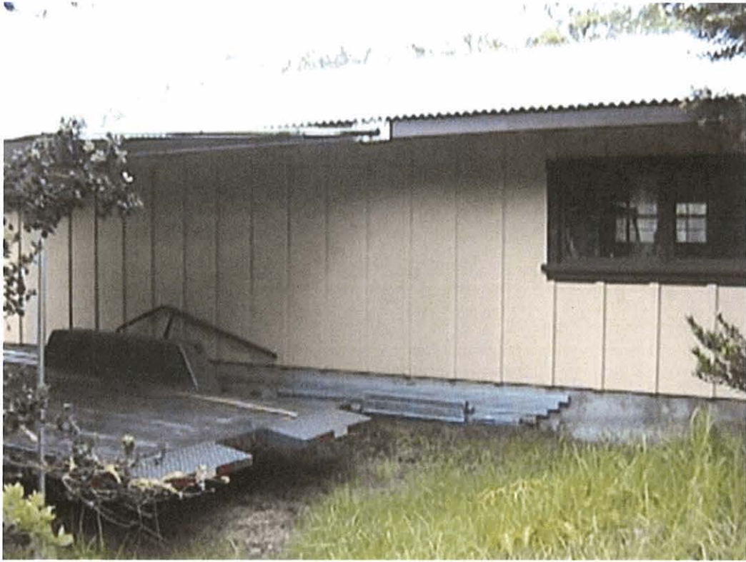
Plate 22. Building #92 with temporary garage, view to the west.
