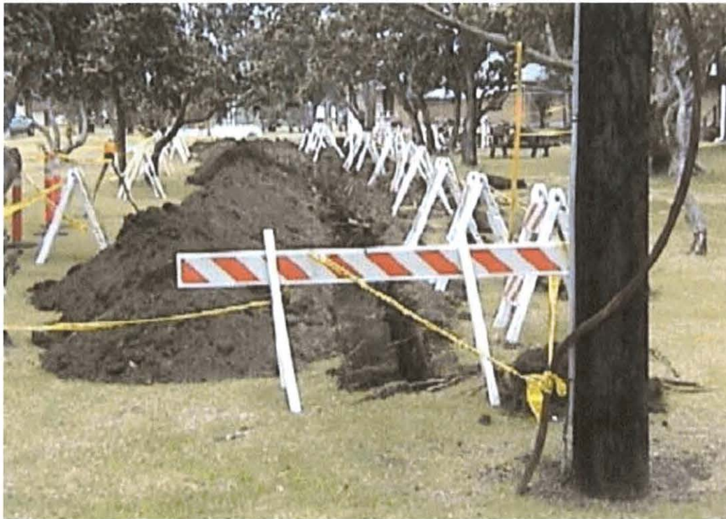
Plate 18. Leg 1 after excavation, view to the east
