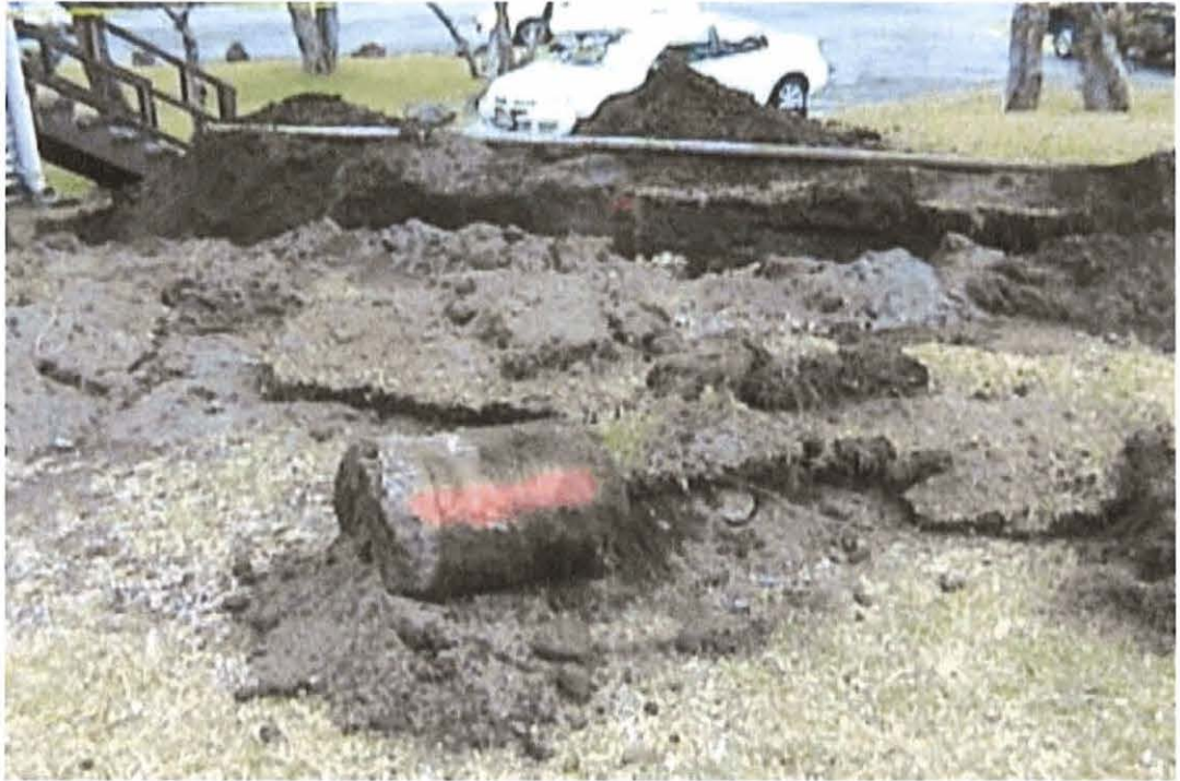
Plate 19. Leg 3, concrete post footer removed by backhoe, view to the north..
